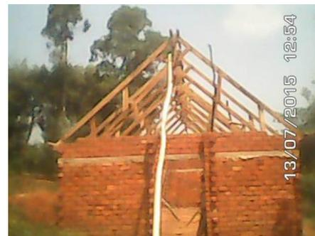
This will be the first church in the Eglise Catholique Anglicane du Congo to be constructed from 'brique cuite' – brick that has been fired in a kiln, and so can withstand heavy rains. As the photographs show, the roof frame is built: now we need money for the roofing sheets! They cost approximately \$15 - \$20 per 4' x 8' sheet.
